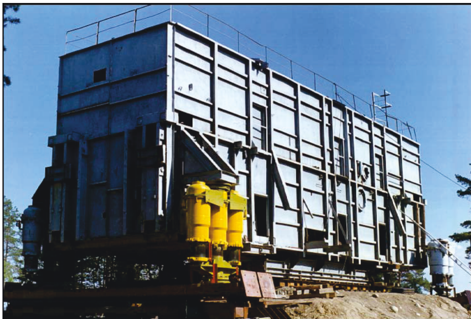
Figure 2.2. Shock-proof object with shock-absorber units.
