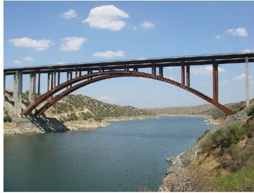
Figure 1. Alconetar Viaduct Bridge (Sánchez Corriols 2015).
