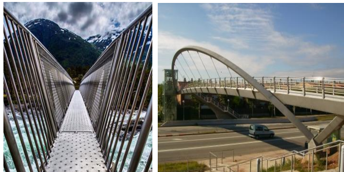
Figure 2. Two examples of bridges using duplex EN 1.4162. Left: Sant Fruitos Bridge; Right: Likholefossen Bridge.
