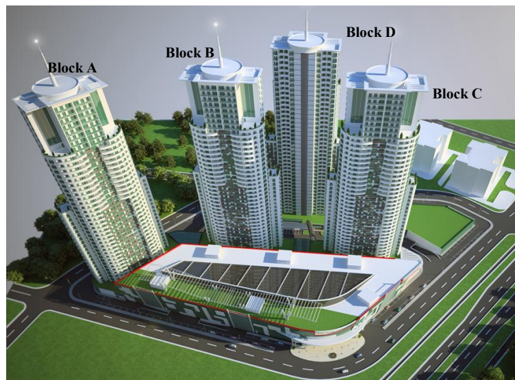
Figure 1. Blocks of the “Cevahir Sky City” residential complex.
