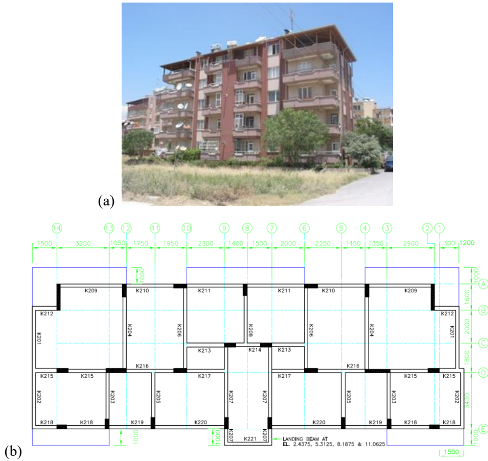
Figure 7. (a) General view of the existing RC structure, (b) Typical floor plan for the upper stories. (Abrahamczyk, 2014).
