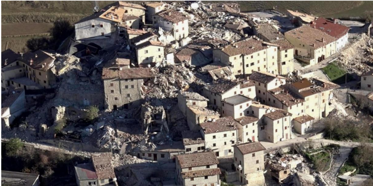
Figure 11. Post-earthquake damaged buildings, Norcia region, Italy. ( http://www.blueseis.com/single-post/2016/12/06/Norcia )
