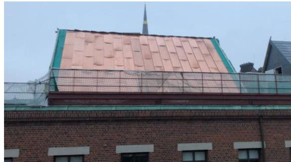
Figure 3: Copper-look roof element (Source: Eckpack GmbH)
