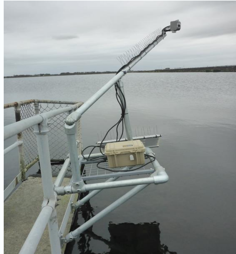
Melbourne Water Treatment Ponds, Werribee
