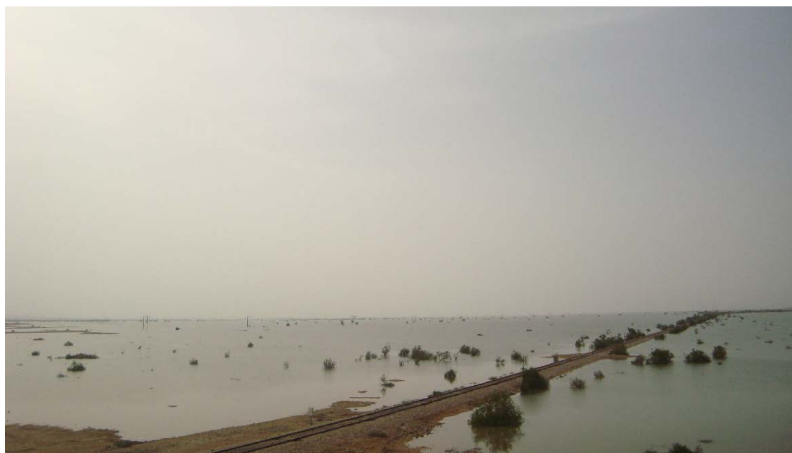
THATTA DISTRICT: The railway tracks of Aamri Station is submerged and not recommended to be used. (WMC)
