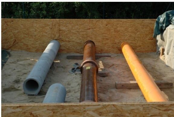
Figure 7: test bed with concrete, stoneware and plastic pipes before embedding them in sand.
