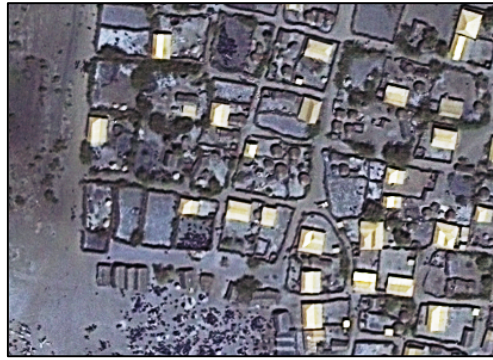
Figure 2.9. A segmentation scenario where the object of interest could be buildings of vastly different spectral and geometric characteristics.
