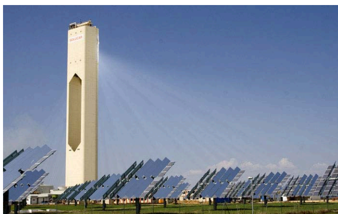
Figure 8: The 11 MW solar heat power plant Planta Solar 10 , Seville, Spain. [14]
