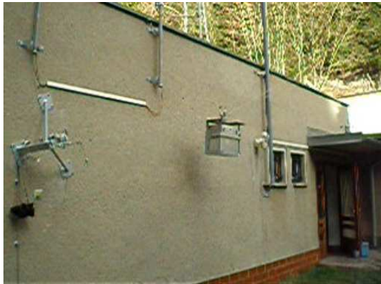
Figure 3.13: Gravimeter lift: lower station in the valley at the observatory building.
