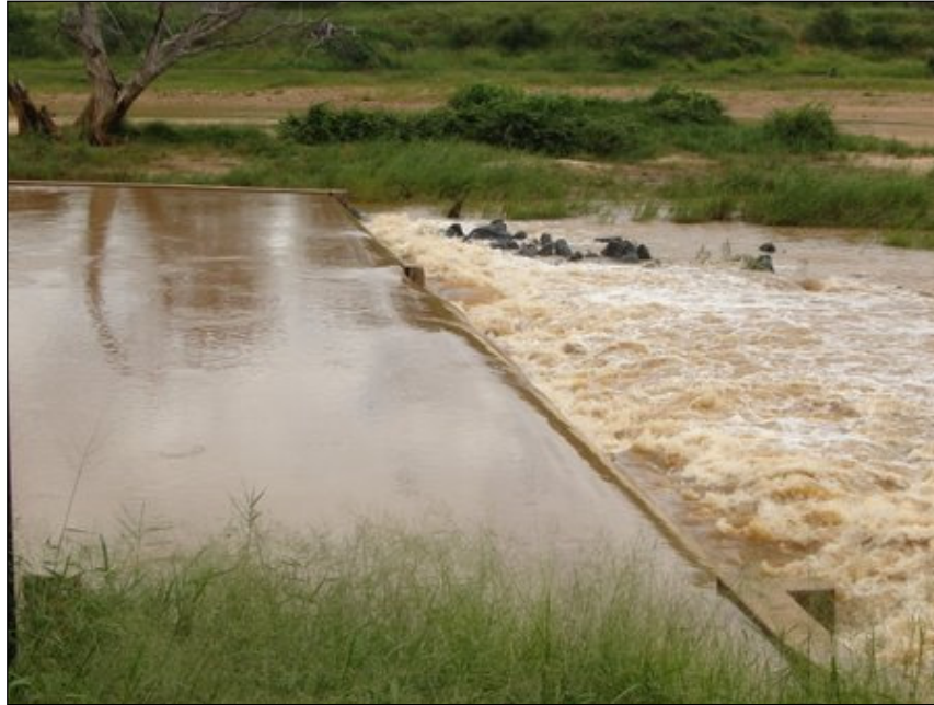
Figure 4-7: The Gauging Station Letaba Ranch (Photo: Scheffler, March 2006)
